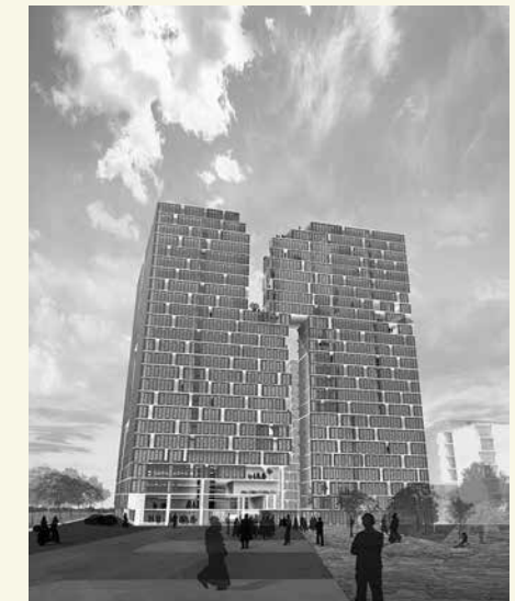
The Tellapur O2 (2008) is a concept for a building in Hyderabad, India, and is part of Studio Gang's growing international portfolio. The project builds on the facade concept for the Brick Weave House, but translates it into a different scale and cultural context by incorporating self-shading techniques from Indian haveli dwellings.
