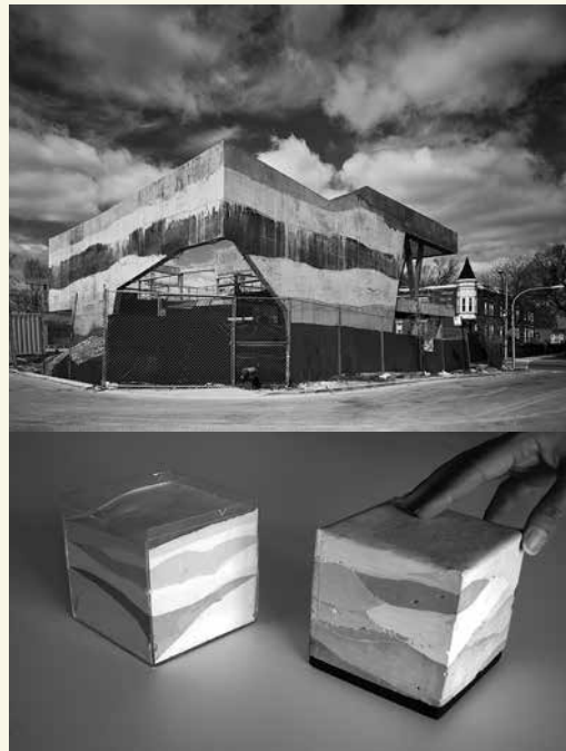
The goal of the SOS Children's Villages Lavezzorio Community Center (2008) is to bring foster-care families and the larger community together under one roof. The center was largely built with in-kind material donations. As a result, some of the exterior walls were poured with various mixes of concrete. Studio Gang used plaster models to develop the concept and communicate it to the contractors. Photograph (above) by Scott McDonald © Hedrich Blessing.
